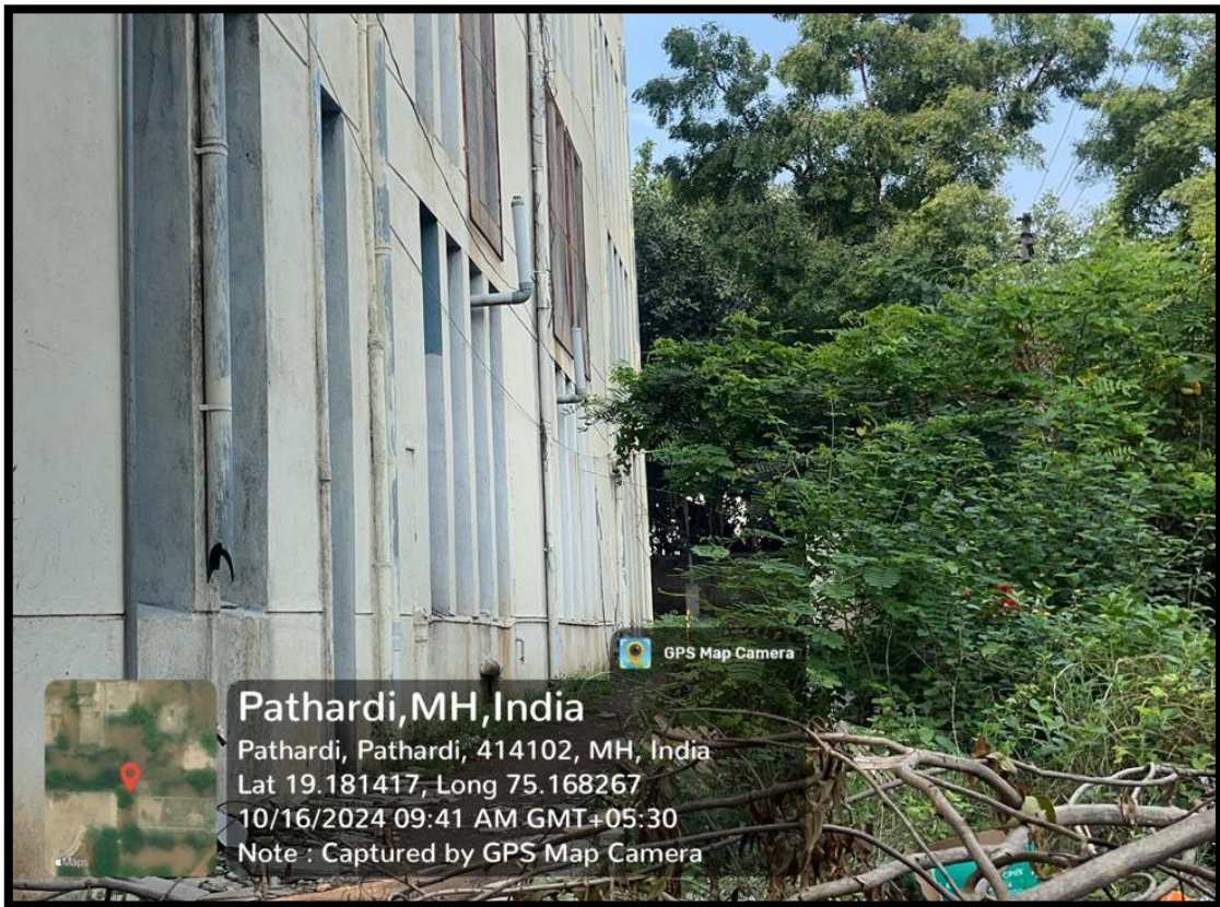
Rain Water Harvesting system at College Campus
