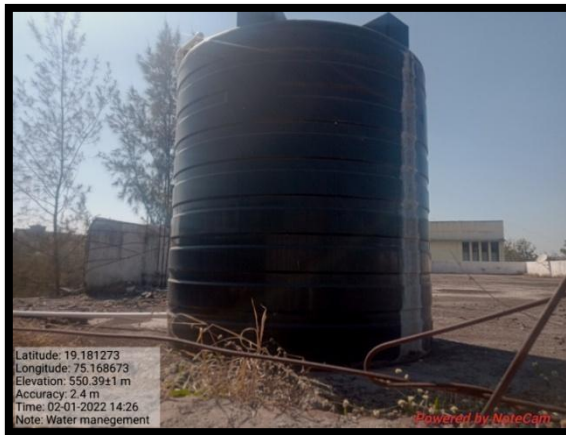
Water storage tank and water distribution pipe system.
